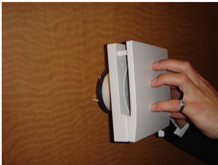
Figure 6: Passive air inlet - Ventilation air can only be introduced into multifamily units through infiltration through exterior walls or directly into the units by ducted supply or passive air inlets - holes in the exterior walls
