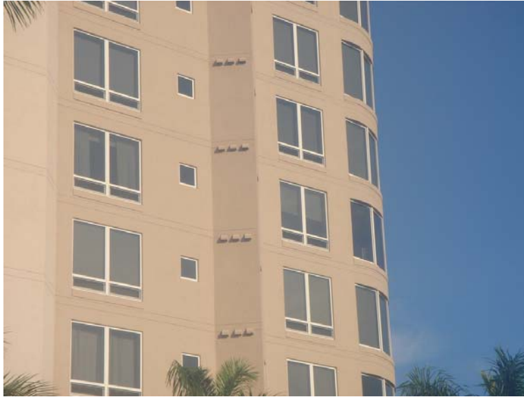
Figure 12: Individual supply and exhaust openings – Multiple exhaust grilles and supply grilles are required
