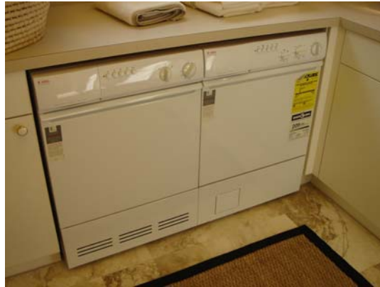
Figure 16: Clothes dryers - Where clothes dryers are installed they should be unvented condensing units – or if vented to the exterior a provision for powered make-up air must be provided
