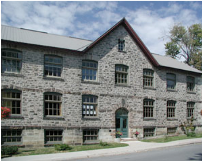
Photograph 5: Big Hygric Buffer—Lots of moisture storage in old mass assemblies constructed from rocks, mortar, bricks and plaster.
