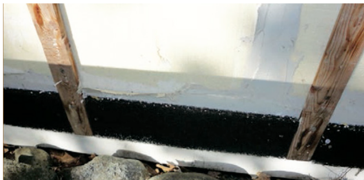
Photograph 9 (bottom): Insect Mesh —Polypropylene mesh acting as an insect barrier is installed between the furring strips at the bottom of the wall. This particular mesh typically is used in attic ridge vents to keep bugs out of roofs.
