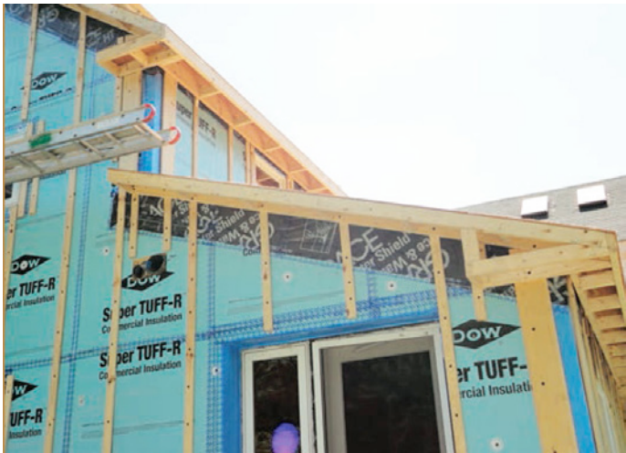
Photograph 14 (top left): Floating Roof —This takes a little bit of thinking to see what is going on. Check out Figure 1 and Figure 2 and then come back to this photograph. The overhangs are structurally sound, they just don't look that way until you understand how box beams work and that the rigid foam is not going to slide down the slope.
