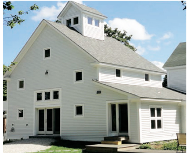
Photograph 14 (top left): Floating Roof —This takes a little bit of thinking to see what is going on. Check out Figure 1 and Figure 2 and then come back to this photograph. The overhangs are structurally sound, they just don't look that way until you understand how box beams work and that the rigid foam is not going to slide down the slope.
