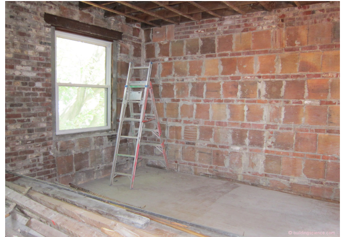
Photograph 2 – Clay Tile: Excellent condition. No large void areas.
