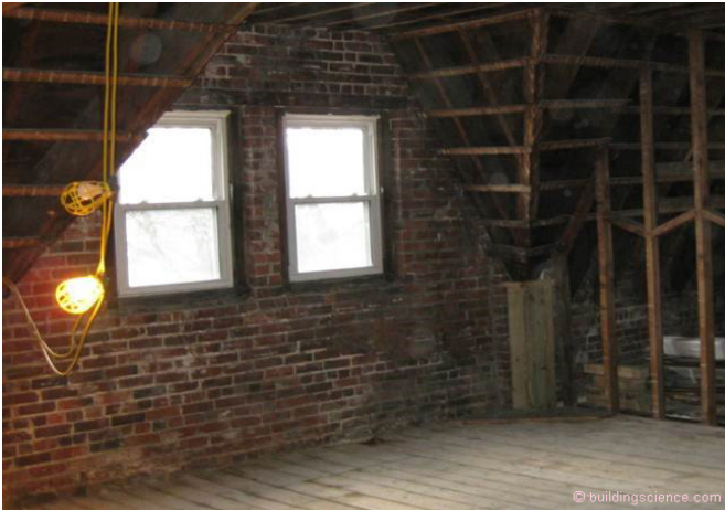
Photograph 1 – Solid Brick: Excellent condition. No large void areas.
