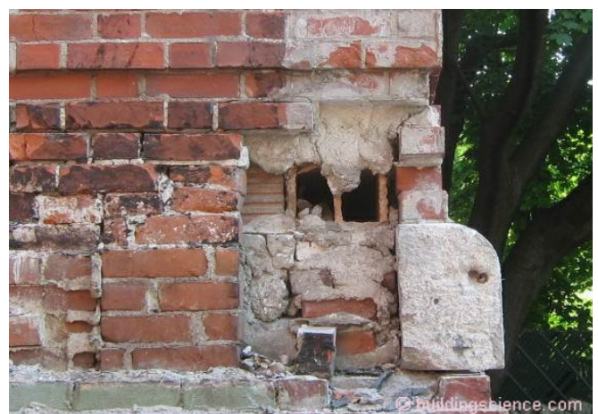
Photograph 4 – Clay Tiles: Clay tiles are hollow. Did I mention that solid mass walls are not typically solid...
