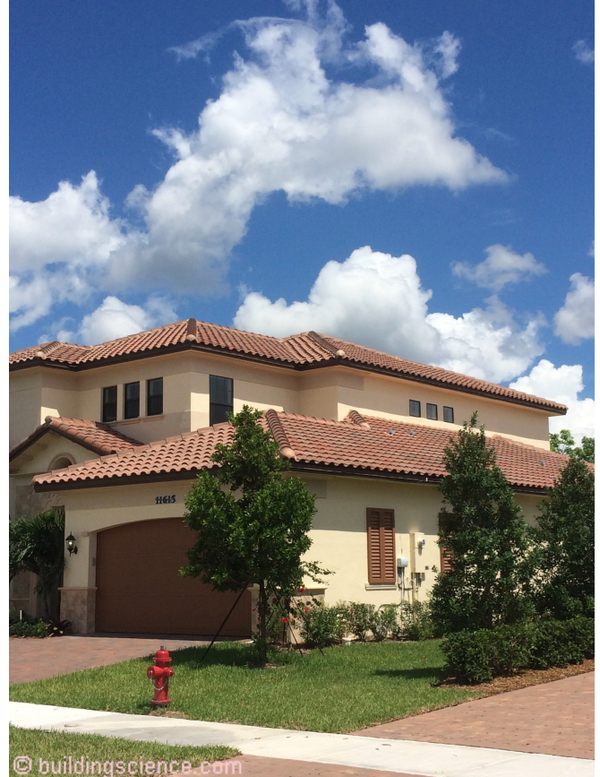
Photograph 5: Tile Roof - Tile roofs are everywhere in south Florida...not so many in south Texas. Tile roofs handle the radiation thing much better than asphalt shingle roofs. With tile roofs dominating south Florida we have “cool roof” technology at its best.
