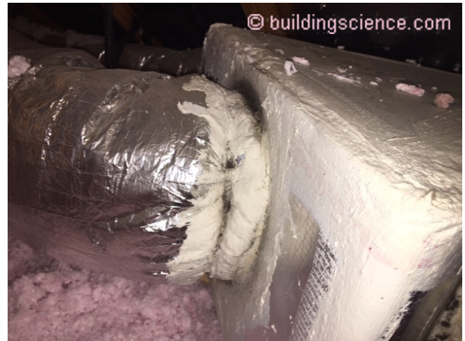
Photograph 3: Mastic - Mold on mastic in a vented attic...a space that is outside the house. Most mastics are “white” in color so you can actually see the mold.
