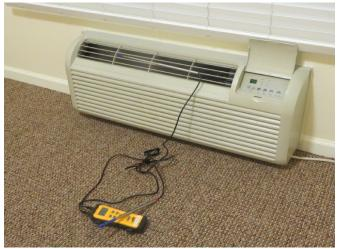
Figure 17: Measuring a PTAC supply and return
