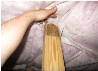
Figure 9: Mold on truss top vertical member
