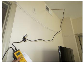
Figure 14: Measuring "split" at supply
