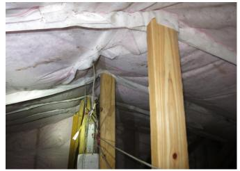
Figure 8: Mold spotting on netting near ridge
