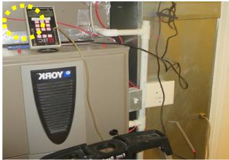
Figure 21: Measuring static pressure
