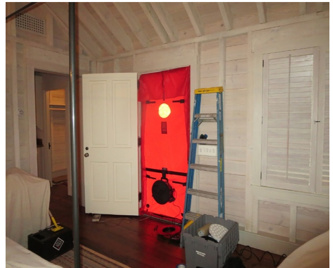
Figure 2: Testing a cottage with a Duct Blaster®
