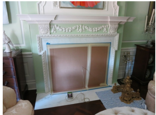
Figure 6: Measuring \Delta P across a fireplace seal
