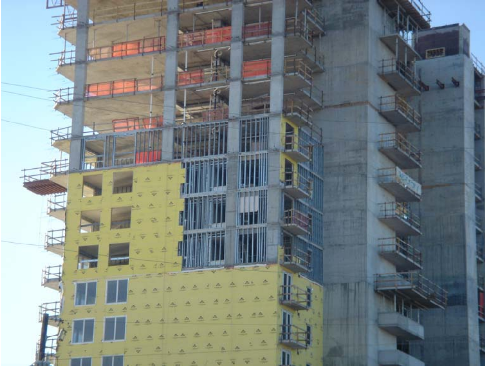
Photograph 6: Non-Paper-Faced Exterior Gypsum Sheathing Over Uninsulated Steel Cavity
