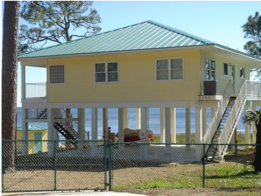
Photograph 2: New Home – Florida Panhandle. "Note the location of the HVAC unit."
