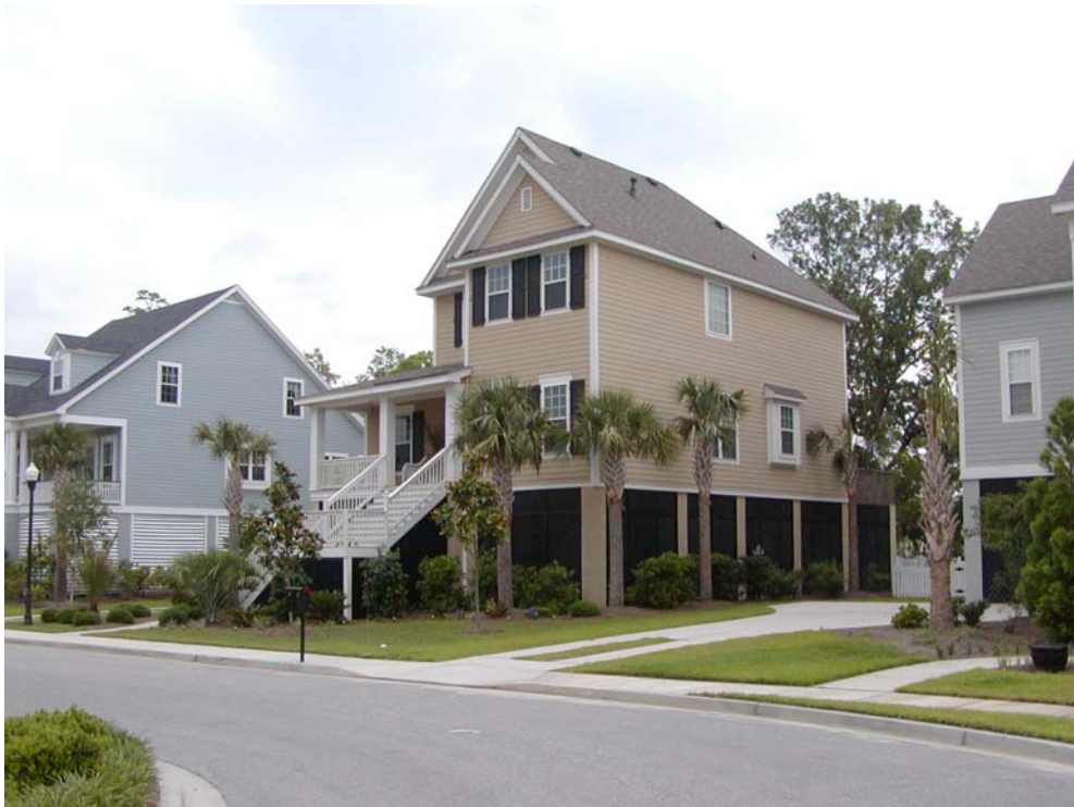
Photograph 1: New Home – Charleston, SC. “First level used for parking, storage and building access.”
