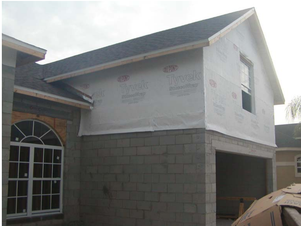
Photograph 5: Residential Rustication in Florida. "The first level is masonry and the second level is wood frame."
