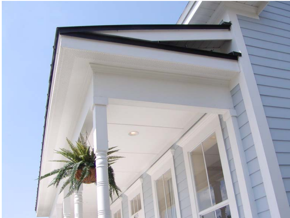
Photograph 8: Look Ma – No Wood. “Non-water sensitive plastic and fiber cement exterior trim and cladding elements installed over a ventilated exterior air space (i.e. cladding is ‘back-vented’).”
