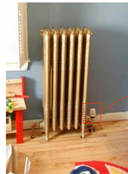
Thermostatic Radiator Valves (TRVs): every radiator its own zone
