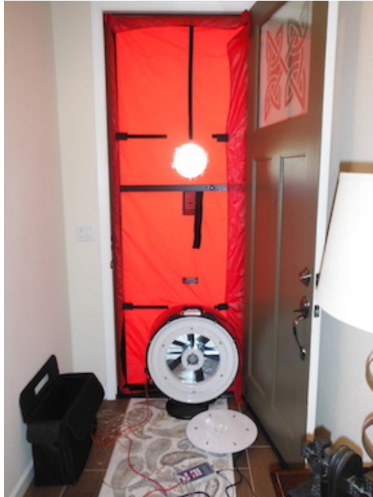
Envelope and Duct Leakage
